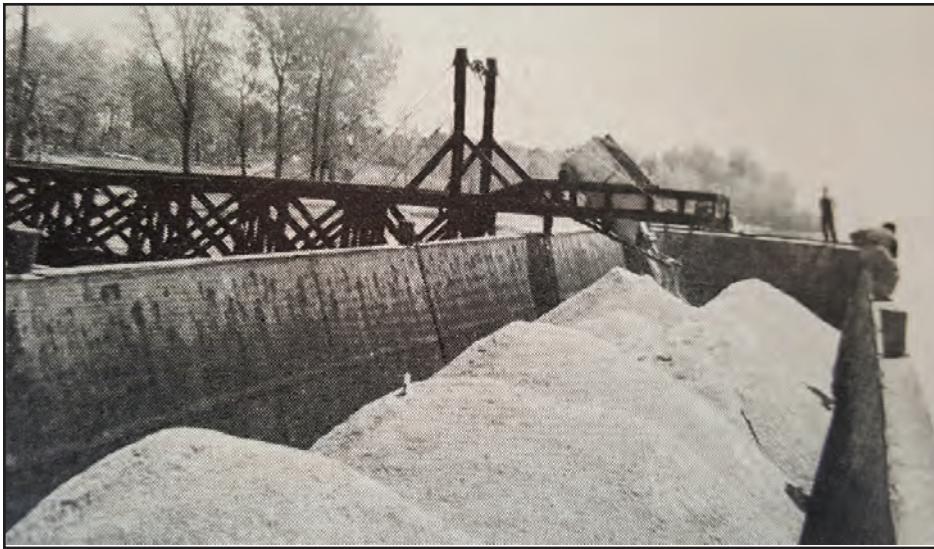
The Crystal Fluorspar Company relied on this Ohio River loading facility to market its product. Barges were capable of carrying up to 550 tons each. This load may be headed to steel mills in Pittsburgh; Granite City, Illinois; Gary, Indiana, or elsewhere. Photo from Mines and Minerals in Illinois, An Industrial Romance, State Department of Mines and Minerals [1945].
